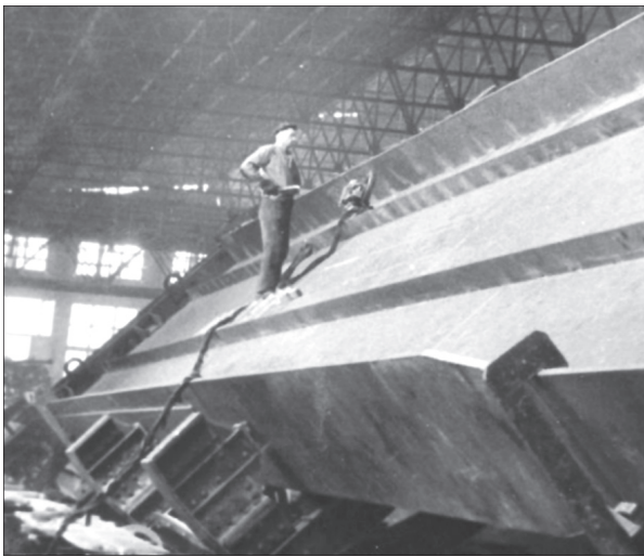
Figure 1. Welding of longitudinal stiffeners and girth welds of the truss [3]
